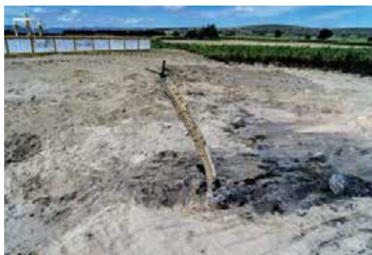
◀ A pipeline in Puebla after it was illegally tapped
